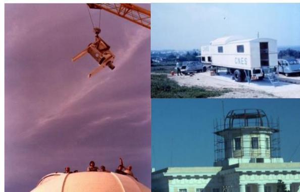
Figure 2. Photographs of the first-generation laser station installed at ROA by CNES, top right; the modifications to the dome for its adaptation to the laser station, bottom right and the final installation on the left in December 1979.
