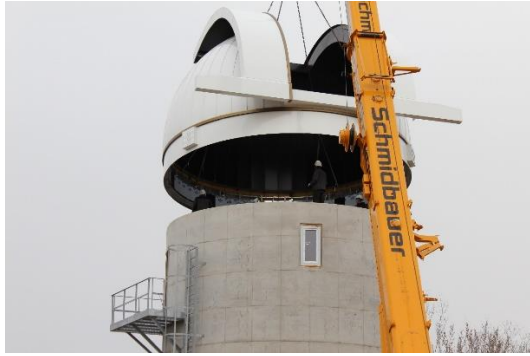
Figure 4. Installation of dome (Gambato) at observatory (Mar. 3, 2021). Image: DLR.
