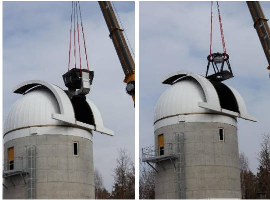
Figure 5. Installation of ASA AZ1750 (Mar. 4, 2021). Image: DLR.
