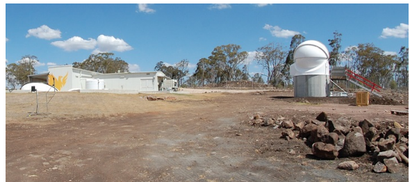
Figure 5. Control building of USQ and telescope station SMART-02-KENT with dome, by courtesy of J. Herzog
