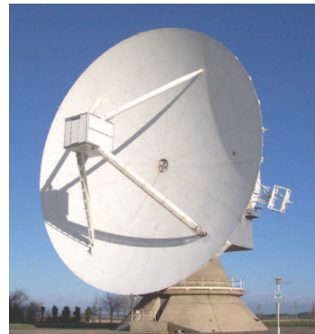
Figure 1. Chilbolton Observatory 25 m radar antenna
