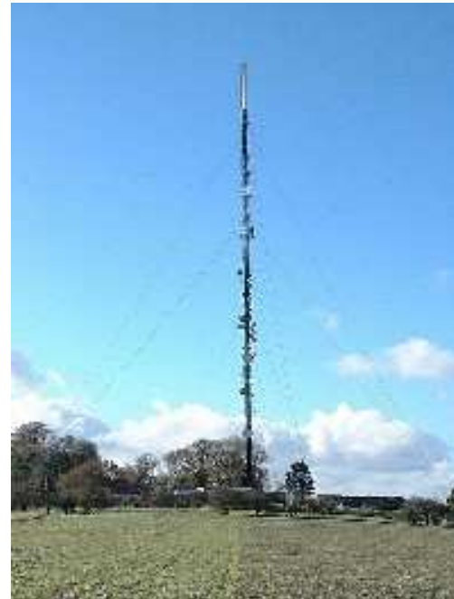
Figure 8. Hannington TV mast, at 22.5 km range from the Chilbolton radar site
