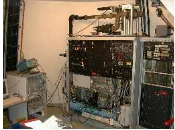
Figure 6. AWS-5 transceiver cabinet installed in the basement of the 25 m dish
