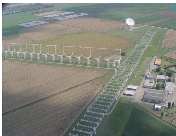
Figure 1. A top view of the Medicina radiotelescopes. In the foreground the T-shaped antenna Croce del Nord. In the background the 32 m diameter parabolic dish.
