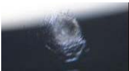
Figure 1. Meteoroid/Debris impact damage on Service Module Window #7
