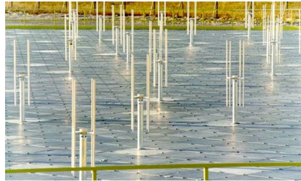
Fig : 6. Reception Antennas
