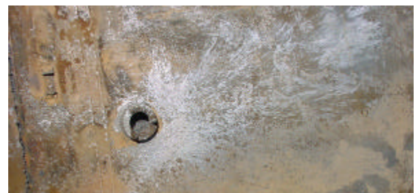
Fig. 3. Metal smears (probably aluminium) visible on stainless steel tank.
