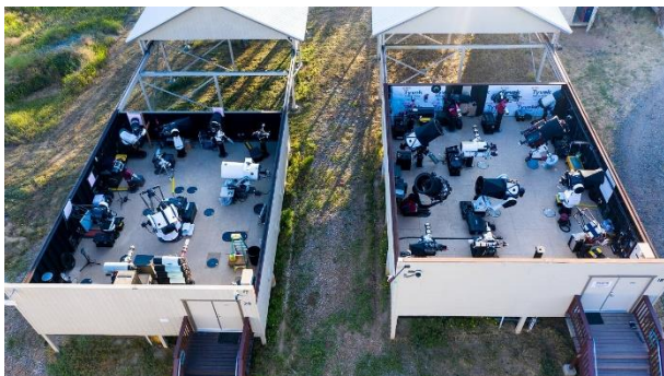
Figure 9. Sliding roof used to host multiple outreach telescopes (credits: Sierra Remote Observatory).
