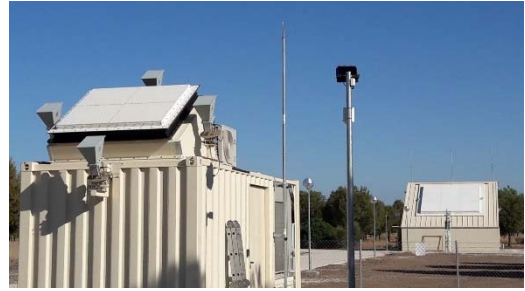
Figure 3. Tx Building (shelter at left site) and Rx Building (right side) of current configuration of S3TSR at Morón AB.
