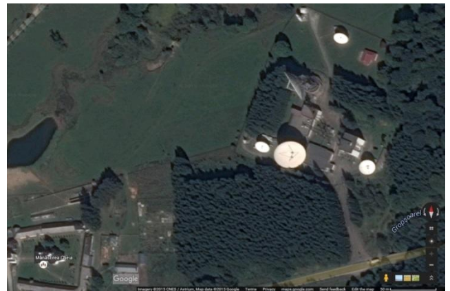
Figure 1. Cheia site and antennas (Google Earth)
